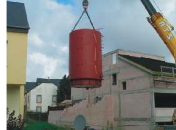
Fig 11: Installation of storage tank
