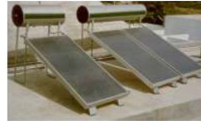
Fig 6: Compact type FPC-based system
