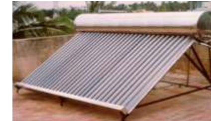
Fig 7: Compact type ETC-based system
