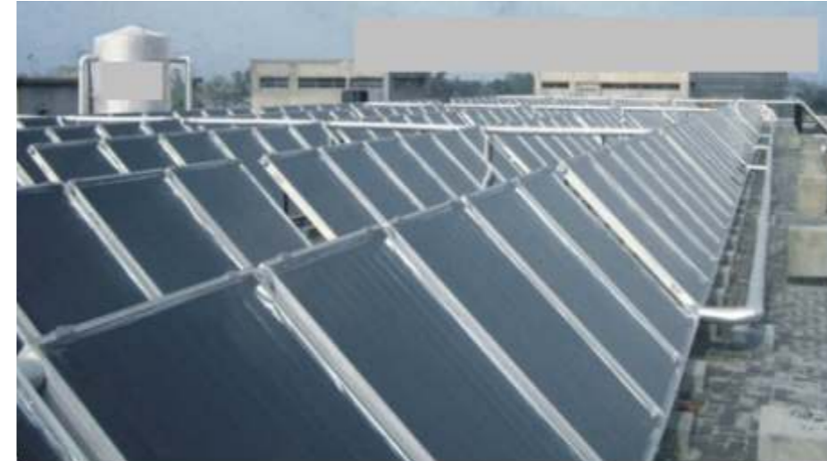
12 lakh Kcal per day system for nickle bath at Kangaroo Industry, Ludhiana
